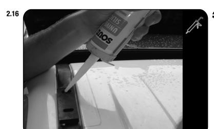
Clean the area around the holes in the vehicle's roof using a rag and denatured alcohol. Place some silicone around each hole in the vehicle's roof.
