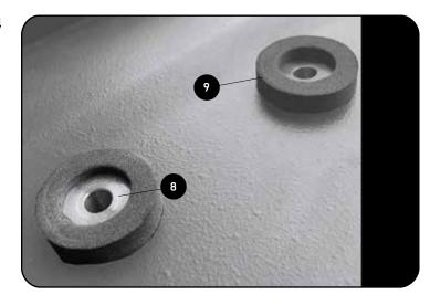
Clean the area around all the 22mm holes drilled in the roof with a rag and methylated spirits/denatured alcohol.
